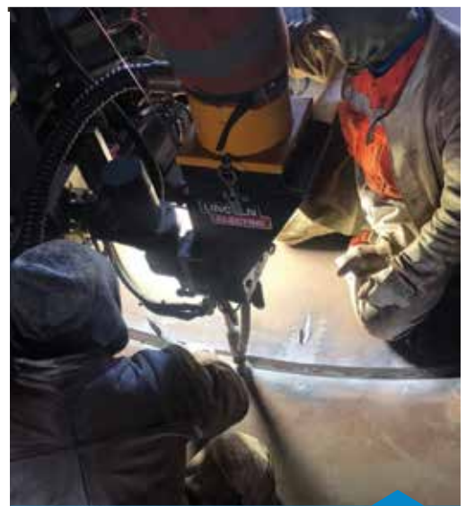
SUBMERGED ARC WELDING (SAW) FOR THE STEEL CASING
